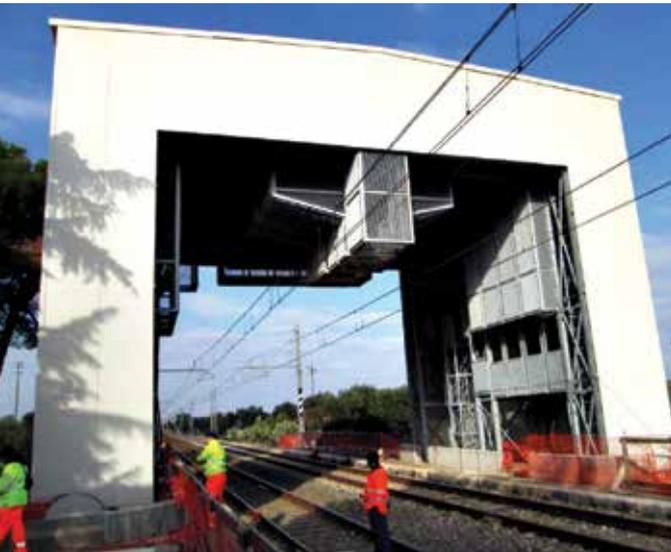
RFI is currently installing its first 'multifunction portals', which will inspect passing trains at speeds up to 300 km/h.
